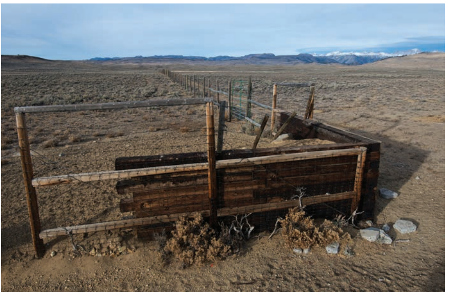
This corner jump-off in an elk fence near the Soda Lake feedground is approximately 5 foot 6 inches tall and rarely used by deer other than mature bucks.
